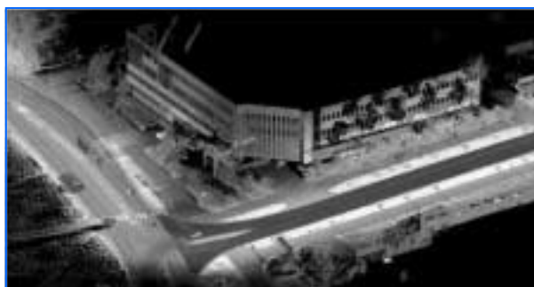
Figure 1. Sky view of a VLS data showing a street corner and office building façade. Courtesy to Antero Kukko, FGI. Acquired by ROAMER.
