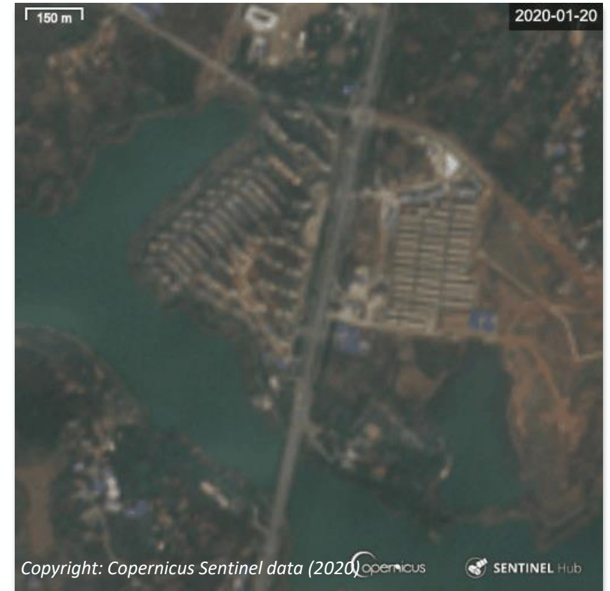
Coronavirus Huoshenshan Hospital construction (Wuhan, China)
